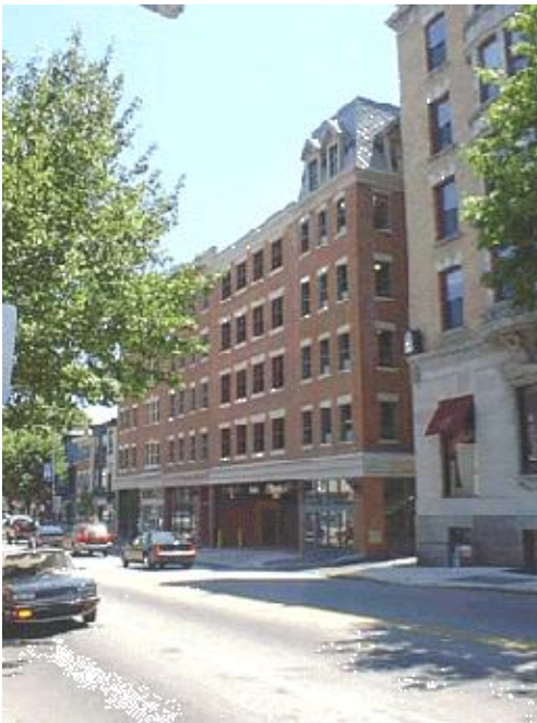
5(b) Bicentennial Parking Garage, West Chester, PA
